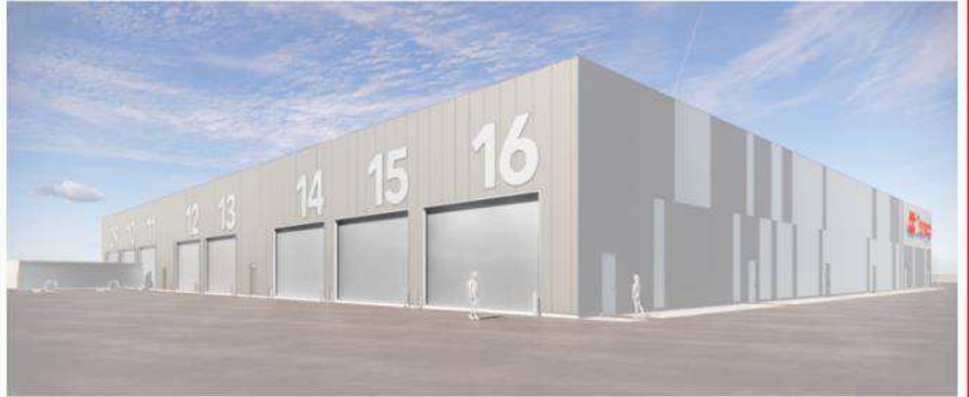
VIEW OF THE BUILDING APPROACHING SOUTH-WEST CORNER
