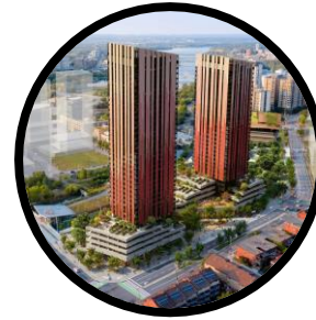
Sewer Energy Exchange Lebreton Flats
